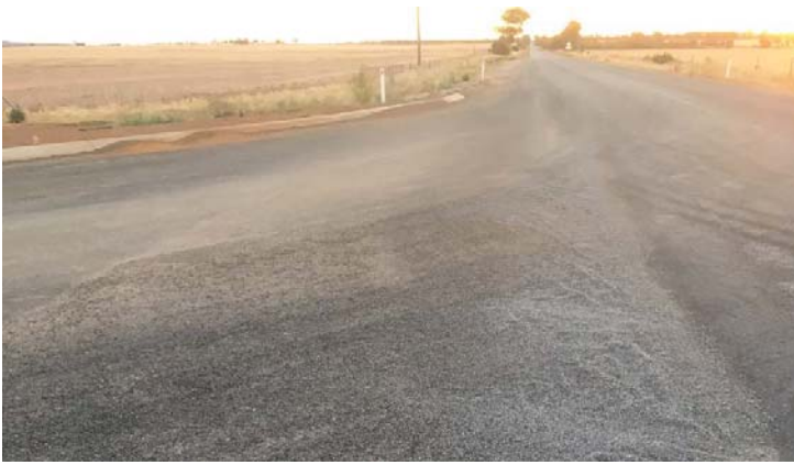
Loose blue metal at intersections to be removed by Works Staff
