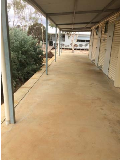
Above: Ablution block
