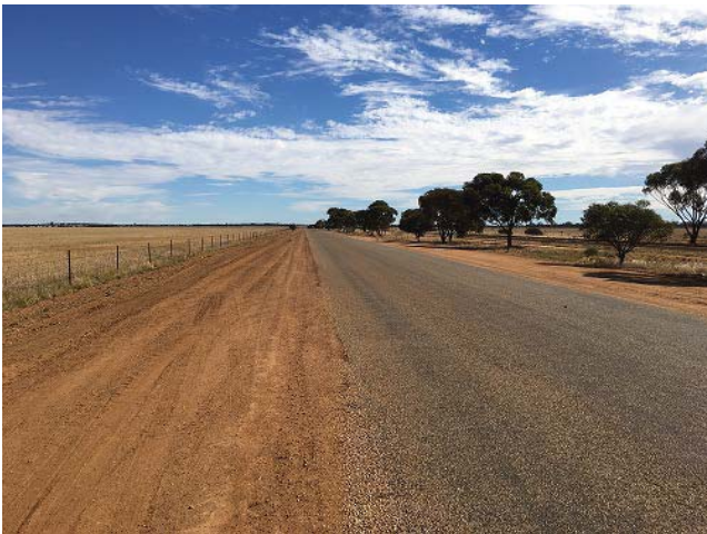
Recently completed shoulder mtce on Koorda Bullfinch Road
